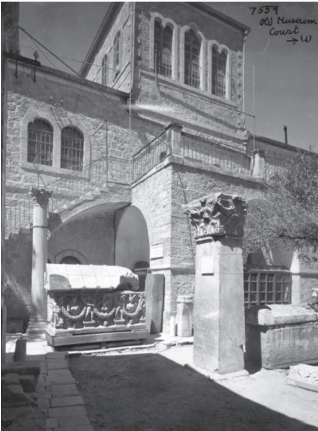
Figure 16: Courtyard and second-story entrance to the Palestine Museum of Antiquities, 1922. Source: IAA Mandate Archives.
